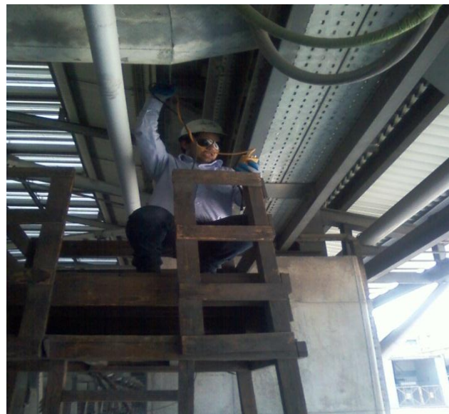
Figure 10DUCT GAS MEASSURING BY FLUKE GAS FLOW METER
